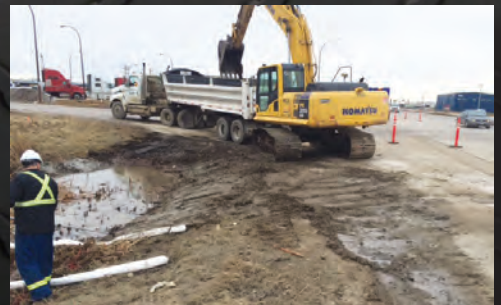
Spill site restoration
